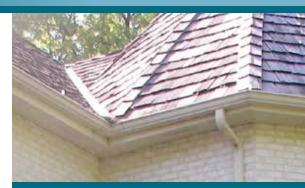
Wood shake roofs with metal valleys are still a challenge even for a 6" gutter.
